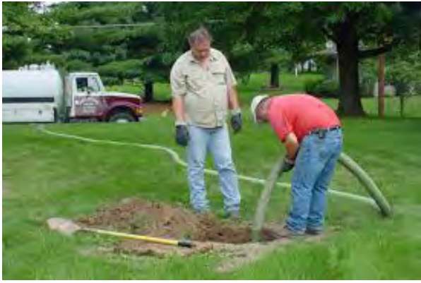
Workers pumping out a home septic tank.
