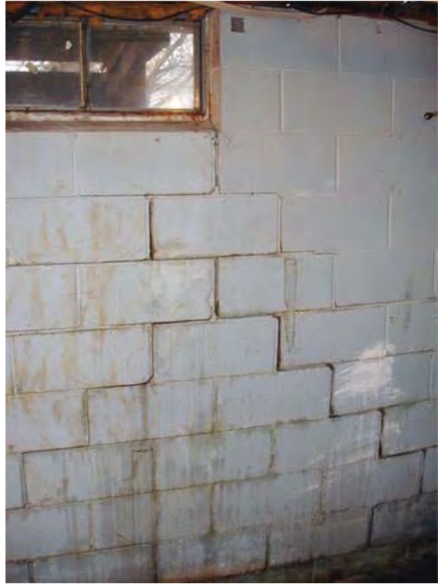
Water can in time heave and damage walls.... actually BOW foundation basement walls
