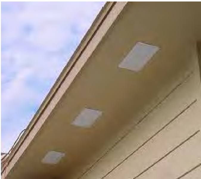
Pictured are some typical Soffit Vent
