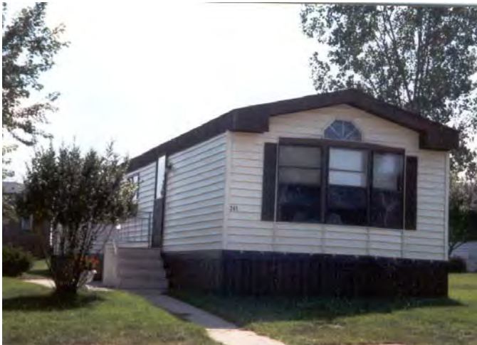
My first house complete with shingled roof, 6" stud walls, and vinyl siding to try to be zoning compliant
