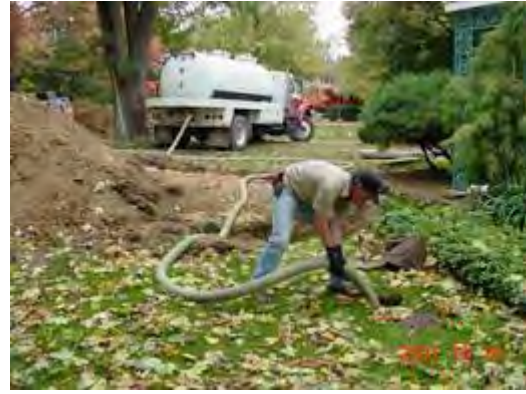
Workers pumping out a home septic tank.
